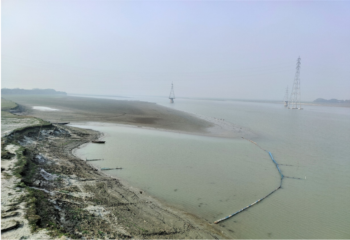
Image 3 : Kosi River As Observed From Kosi River Bridge On 6 th January, 2022
